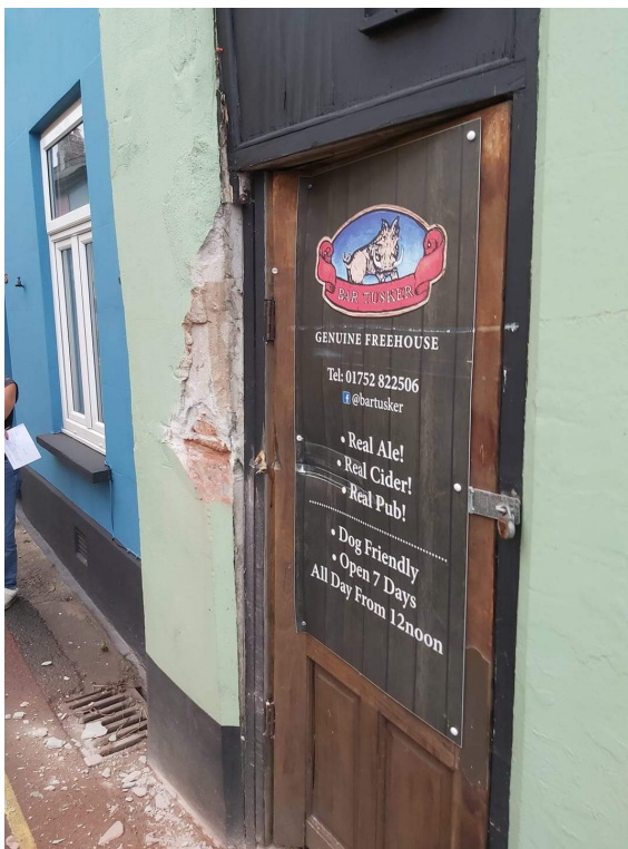
Fig.4 – Damage to a commercial property on West Street caused by an oversized vehicle attempting to navigate the area on 3 rd September 2020.
